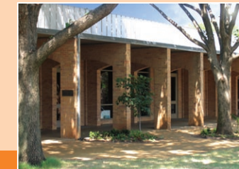
Jerome and Pauline Crossman Hall, 1964 Dining Hall, The Buzz Campus Store Architects: O'Neil Ford and Associates
