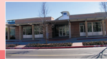
Upper School Addition, 2005 Grades 9 – 12 History & English, College Counseling, US Office Architects: Lake/Flato (design); F&S Partners (project)
