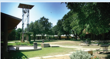
Phillip G. Foote Quadrangle, 1989, 1992 Architects: Ford Powell & Carson; Armstrong/Berger Peter G. Briggs Clock Tower, 2001 Architects: Lake/Flato
