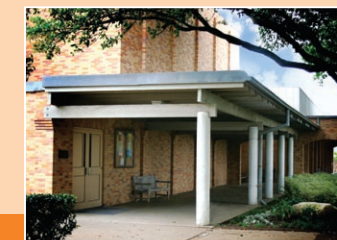
Zale-Fields Theatre, 1974 Architects: Pratt, Box, Henderson and Partners
